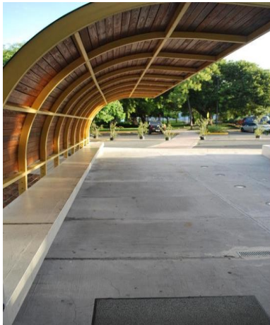
Photo of the emergency exit leading to the University's PG7 parking lot
