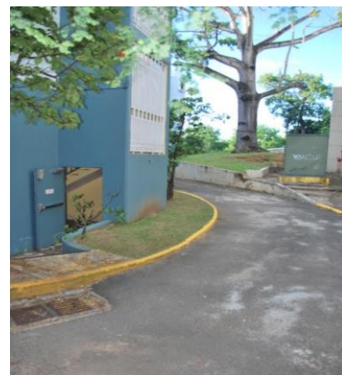
Photos of the south-side emergency exit – Tower B
